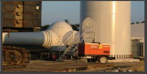
The Equalizer TFA15TI hydraulic flange alignment tool has been developed to aid the alignment of large flanges on the inside of wind turbine tower. This tool will make the installation of wind turbine tower sections simpler, safer and more efficient.
