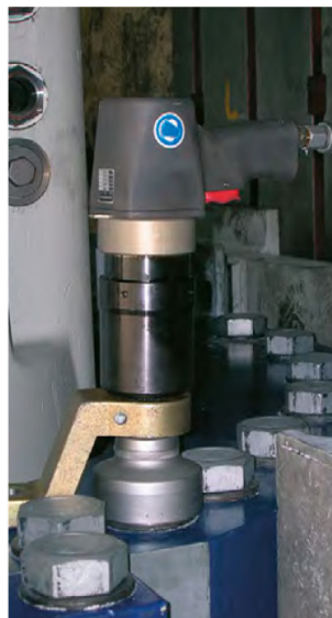
alkitronic® CLD torque multipliers in use (figures on the right). Screw connections at a bolt circle and a diesel unit for large construction machines
