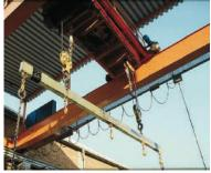
This electrical overhead traveling crane is protected against overload by a PIAB Dynamometer in the hook line anchorage, giving the crane operator the actual load on the hook together with overload warnings and power shunt.
