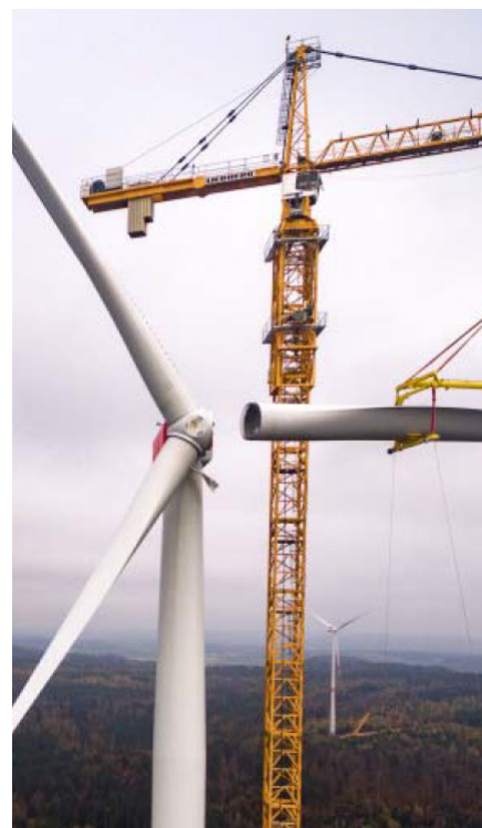
Attaching the leaves. Foto: © Max Bögl Wind AG, photographer: Holger Hessenthaler.
