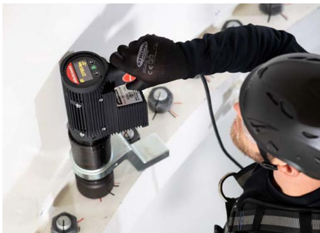
HG 20 AF 60 M36-HV Maintenance on a tower bolt, torque: 2,800 Nm
