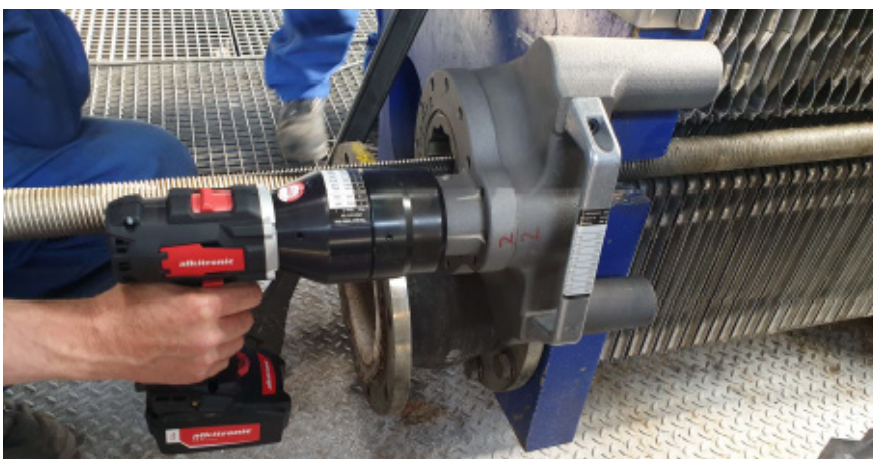
Maintenance of plate heat exchanger Tool used: EAF-SG
