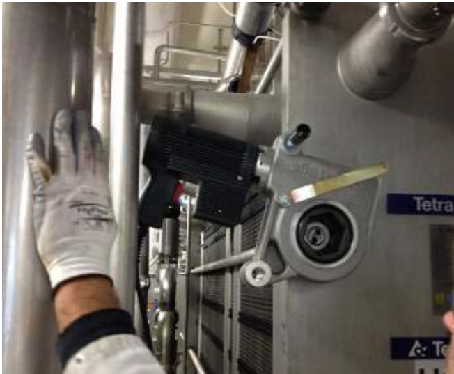
Opening and retightening of the spindles of a plate heat exchanger using alkitronic® EC-R
