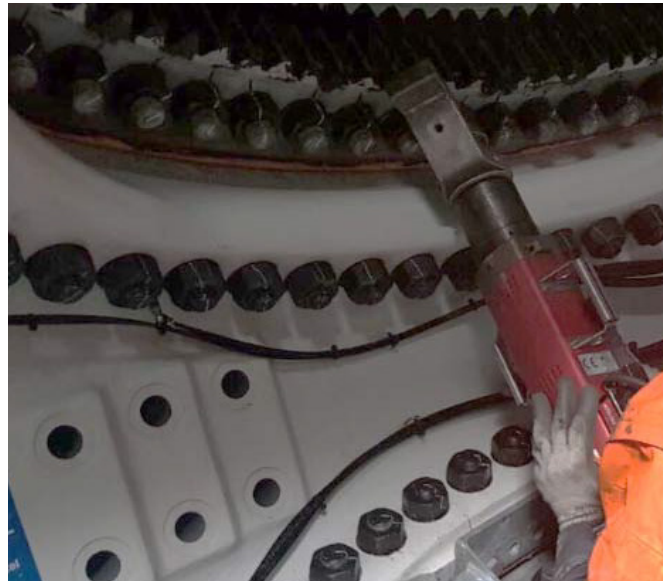
Bolting connections under confined conditions in the rotor housing.
