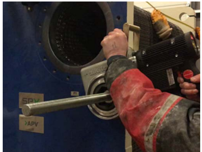
Maintenance and repair of plate heat exchangers with EC-R
