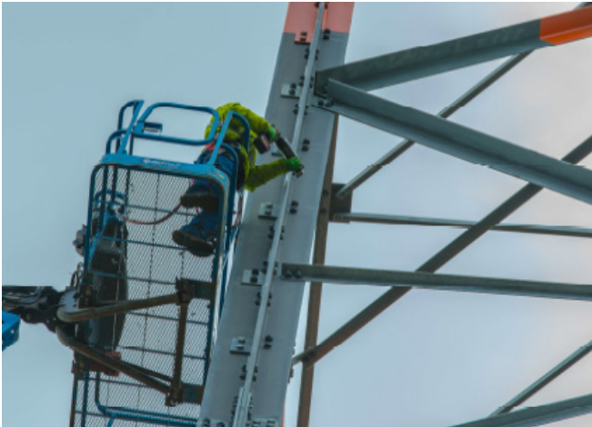
Construction of steel mast for wind turbine using EAF 2/280
