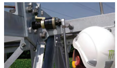
alkitronic® M operating on electricity pylons. Accurate tightening via torque wrench.
