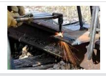
The derail sits on two ties and must be pushed up against the rail head. The tie plates inside the rail will get in the way, so it is necessary to crop the plates close to the base of the rail. The derail base must sit flat on the sleepers.
