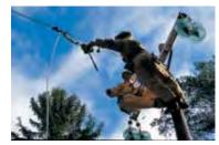
In line construction it is important to control the installed tension of conductors according to type and conditions. For field work light and robust equipment is especially important. The PIAB Dynamometers are used for this duty all over the world.
