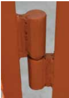
Bullet Hinges, allows 100° Rotation of gate
