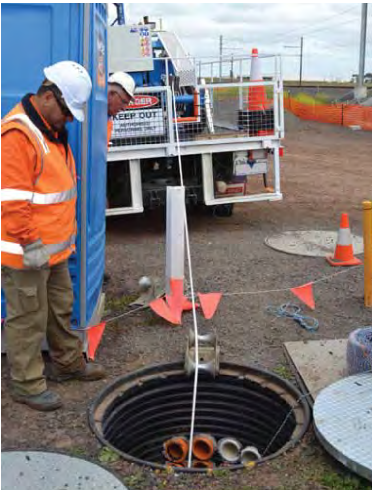
ALWAYS MEASURE CONDUIT ID
