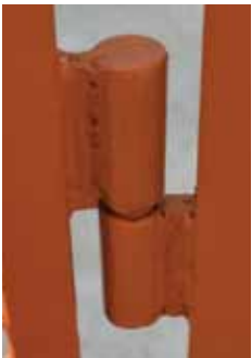
Bullet Hinges, allows 100° Rotation of gate
