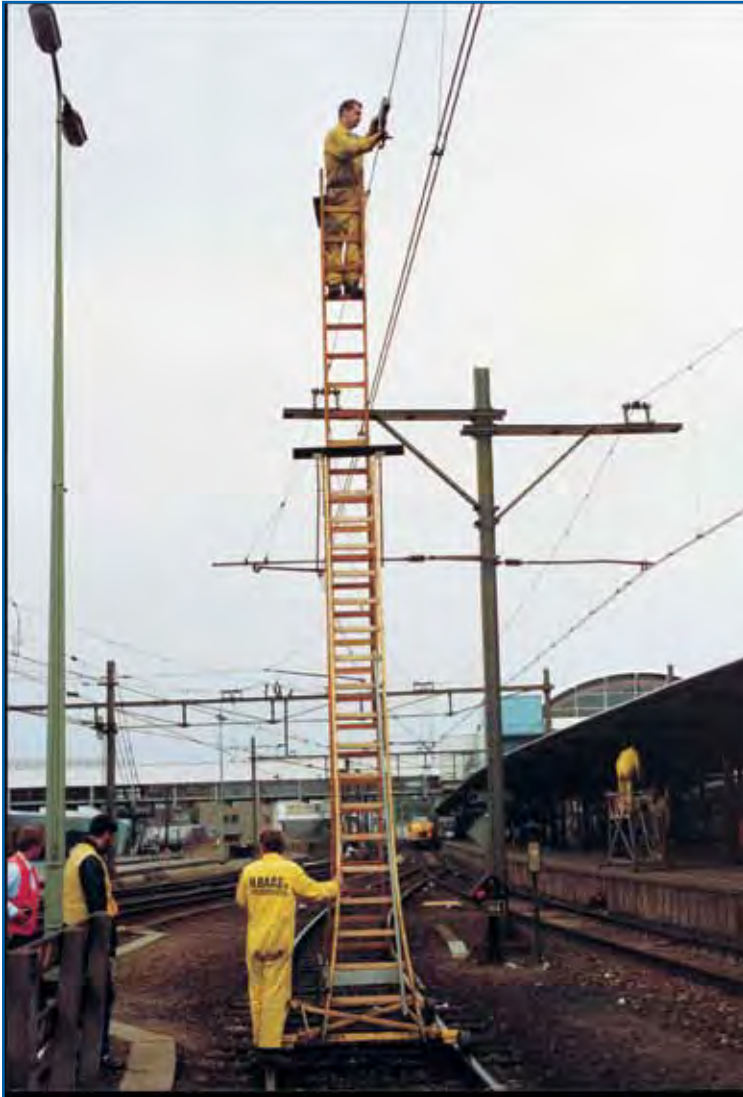
The PIAB RTM 20D is in use when installing/inspecting suspension and catenary ropes.
