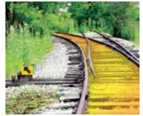
Track Switch Safety
