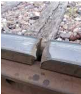
Inspect Your Track
